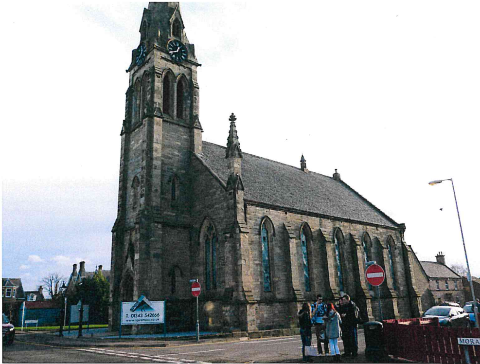
Above: 'SpireRoxx' Rock Climbing Gym, formerly Elgin South Parish Church, 27 Moray Street, Elgin
