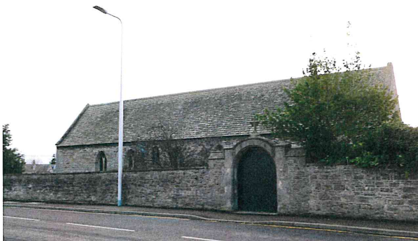
Above: Greyfriars Convent from Greyfriars' Street
