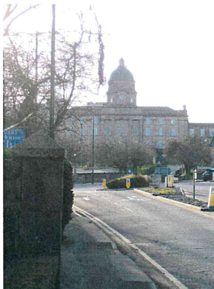
Above: Dr Gray's Hospital from the High Street
